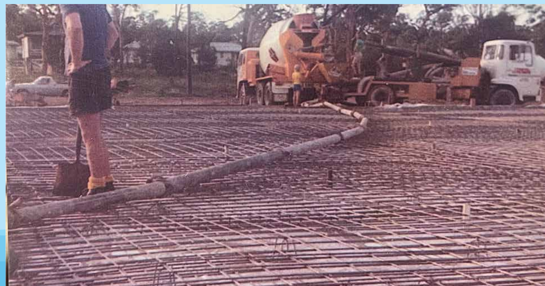
Pouring the concrete slab
