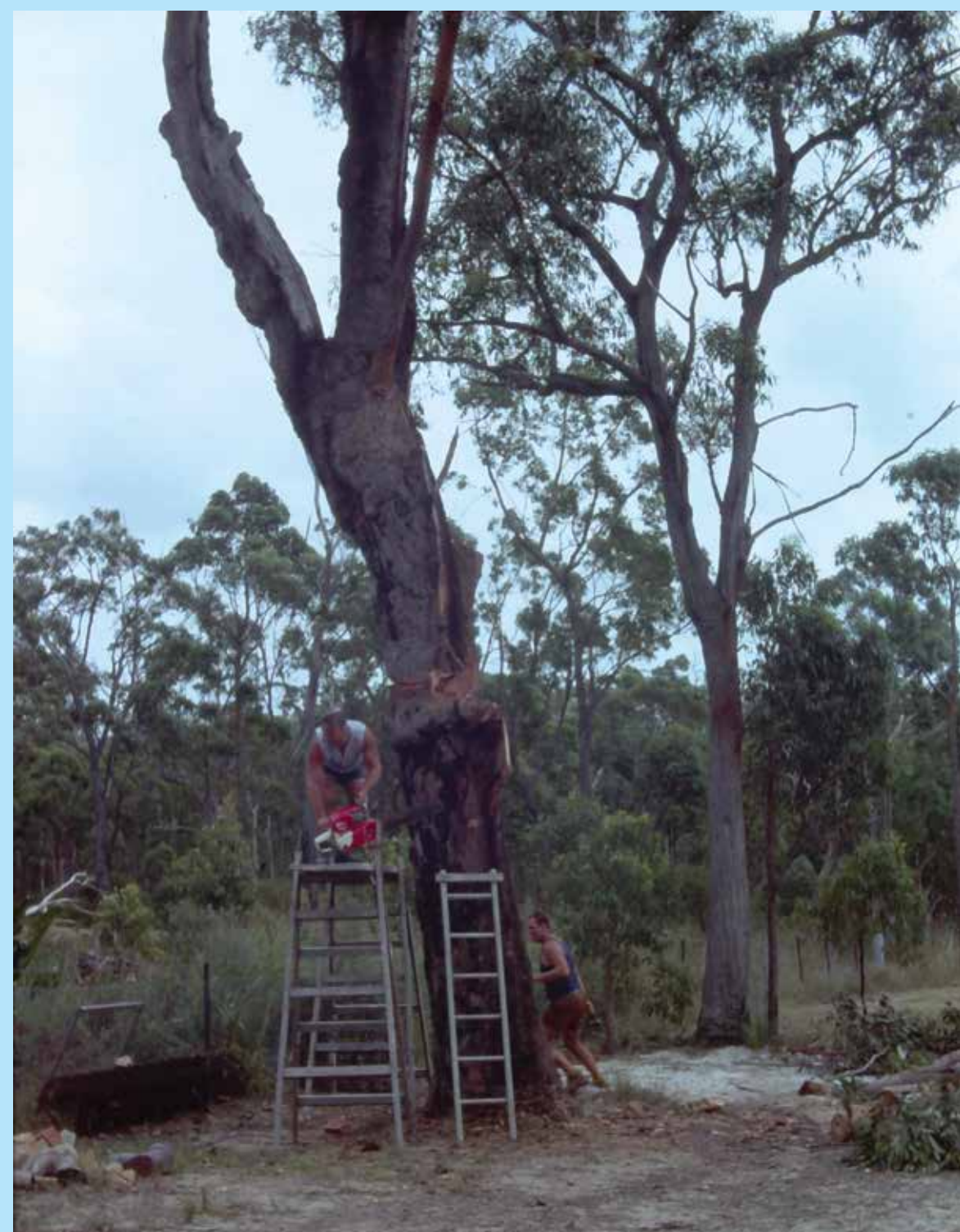
Clearing the site, stump would have been dynamited
