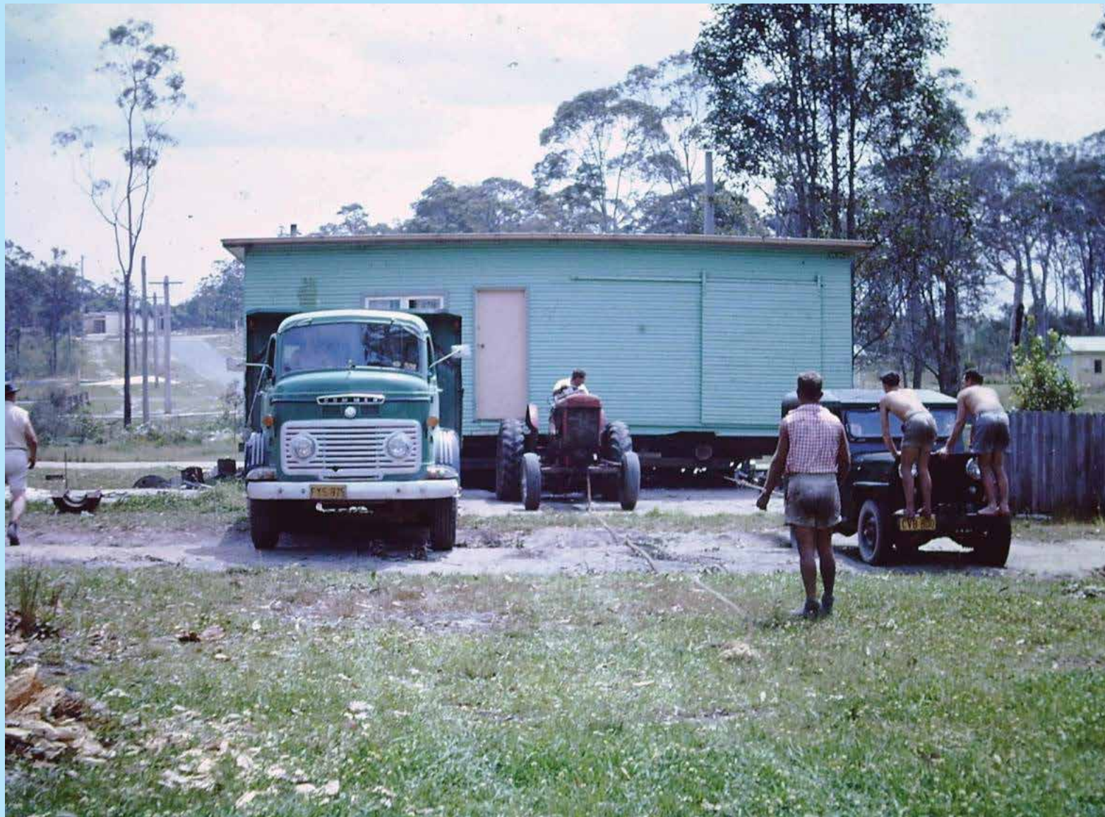
The shop being placed on site
